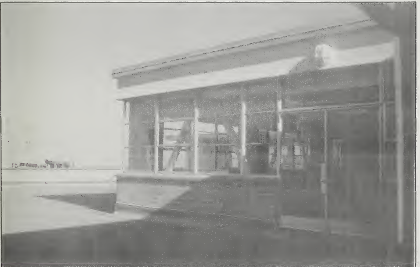
Figure 45 - Penthouse, North Facade
